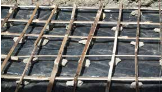
Figure 2: Bamboo splints used as reinforcement for a concrete floor slab.
