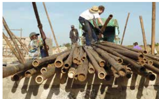
Figure 1: Unloading indigenous Kenyan bamboo on site near Nairobi.
